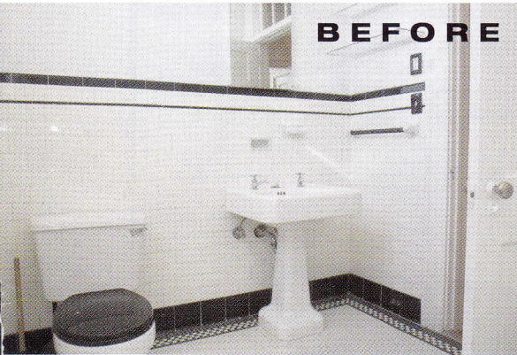
The bathroom underwent considerable alterations, among them replacement of aged subway tiles with white beadboard along the lower half of the walls.
