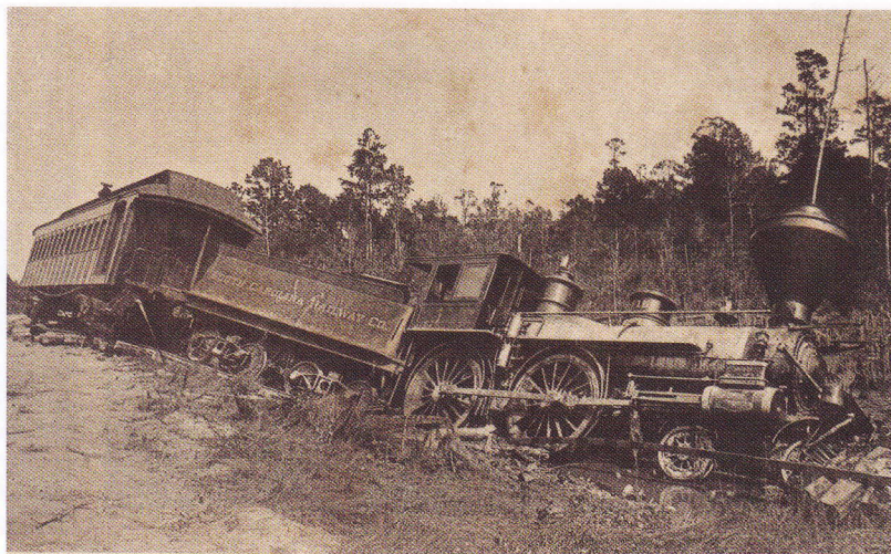
Rolling stock such as this passenger train operated by the South Carolina Railway Co. were derailed, both by the earthquake itself and by dislocated tracks.
