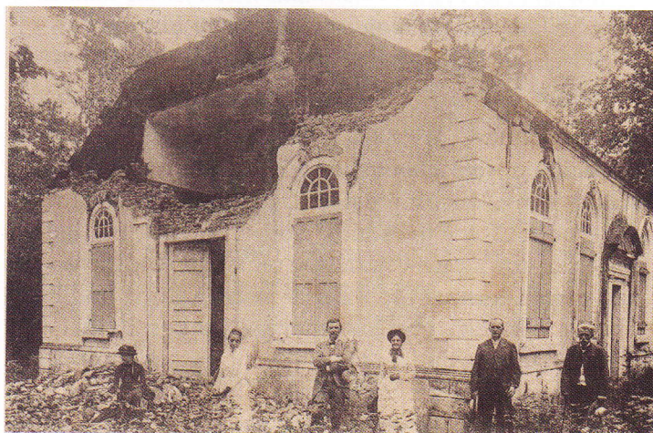
Goose Creek residents pause amid the rubble of St. James Episcopal Church, which was caved in by the force of the earthquake.
