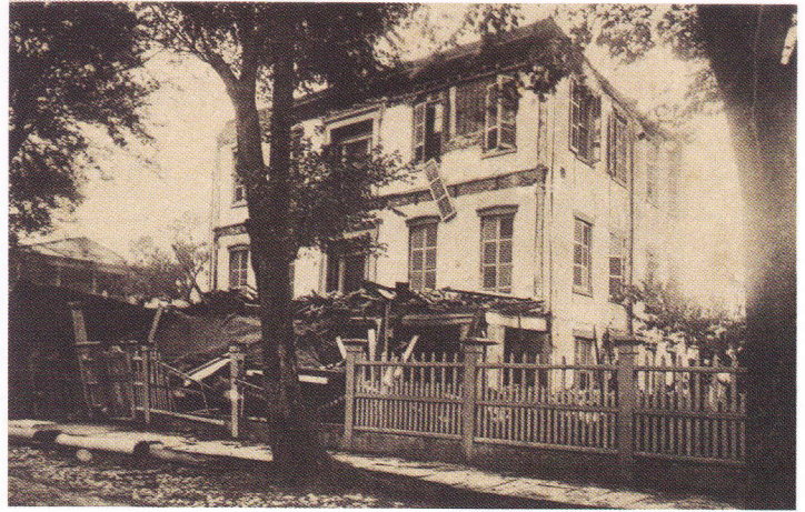
This house on Beaufain Street sustained damage to the piazza and top floor. Today many buildings boast earthquake rods.
