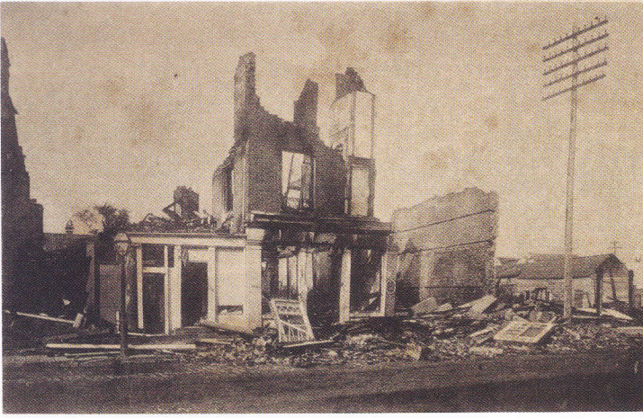
Shortly after the earthquake struck, fires ignited by fallen lamps and candles roared to life. One such fire gutted these buildings at the intersection of Warren and King Streets, near Marion Square.
