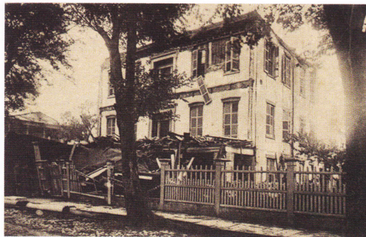
This house on Beaufain Street sustained damage to the piazza and top floor. Today many buildings boast earthquake rods.
