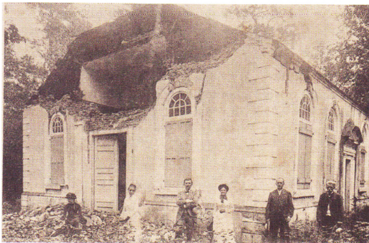
Goose Creek residents pause amid the rubble of St. James Episcopal Church, which was caved in by the force of the earthquake.
