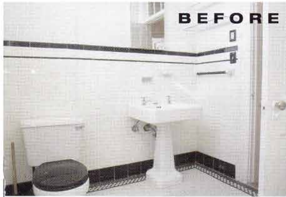
The bathroom underwent considerable alterations, among them replacement of aged subway tiles with white beadboard along the lower half of the walls.
